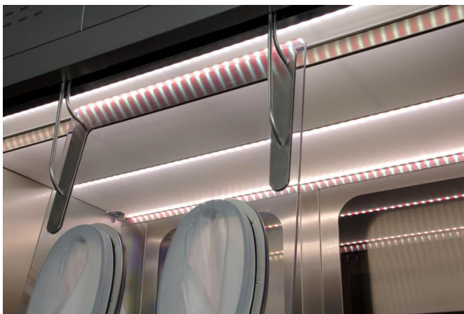
Coloured LED lights signal the operating state of the system and warn of malfunctions.
