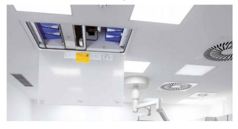
Vindur Top from Weiss Technik has clear operating and maintenance advantages: All of the built-in parts are easily accessible from below, which enables simple and quick replacement of filters and other components.
